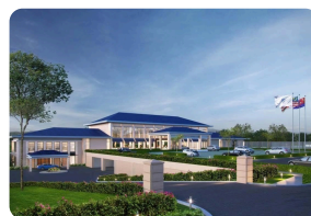
CLUBHOUSE UNDER CONSTRUCTION
