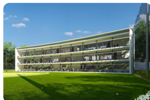
DRIVING RANGE UNDER CONSTRUCTION
